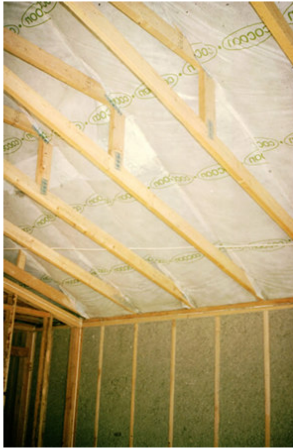
Photograph 3: Netted Cellulose – Air and vapour permeable insulation in hot-dry climate
