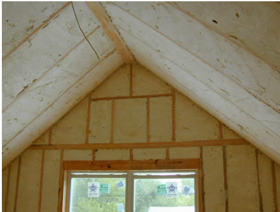
Photograph 2: Spray Foam Insulation
