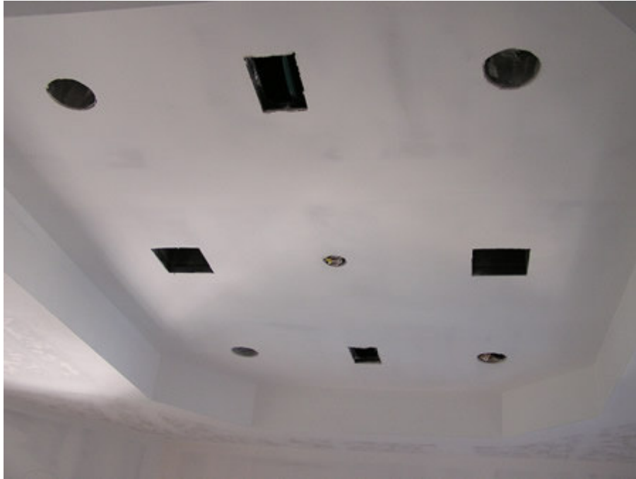
Photograph 1: Ceiling Penetrations – “Swiss Cheese Services”
