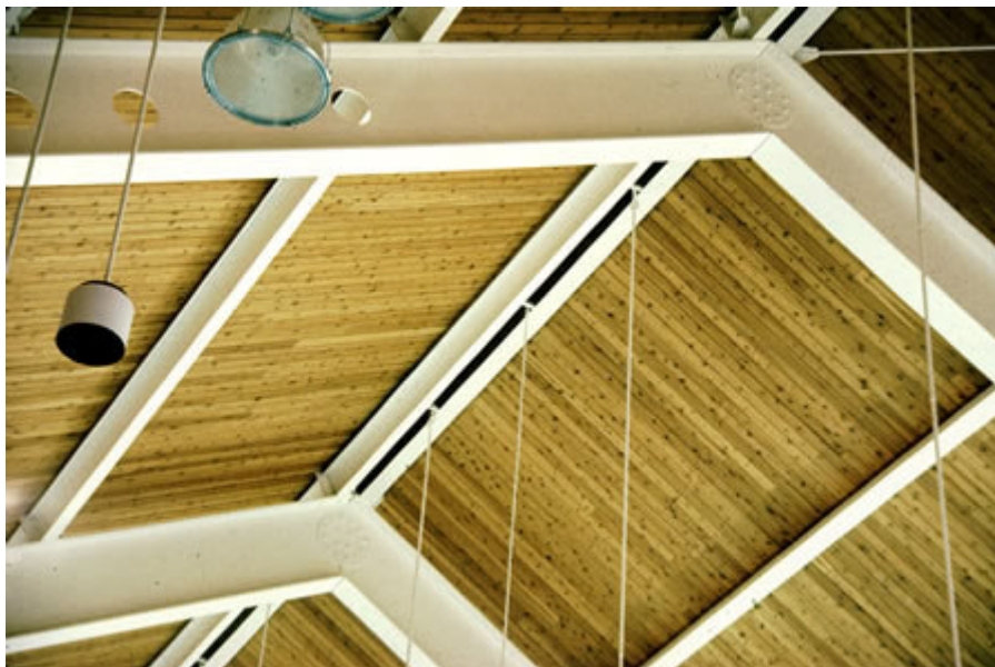
Photograph 4: Compact Roof For Pool Enclosure
